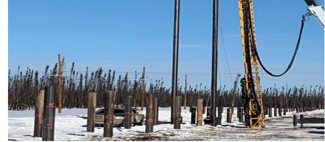
Pile Foundation Construction at Wellpad
