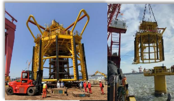
Key R&D products: Pile-based single-point mooring system
