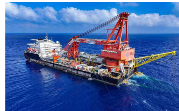
The subsea pipeline laying site of the "Offshore Oil 202" vessel
