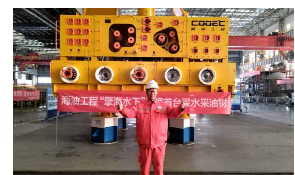
China's first 2,000-meter-class deepwater subsea tree successfully installed
