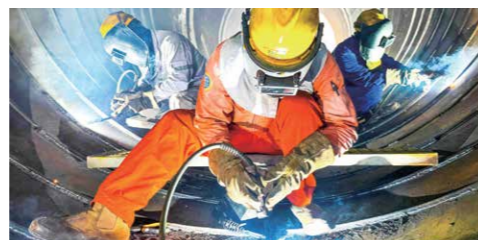
Strict control of welding quality
