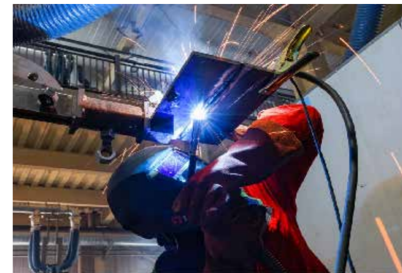
Contestants performing welding on-site
