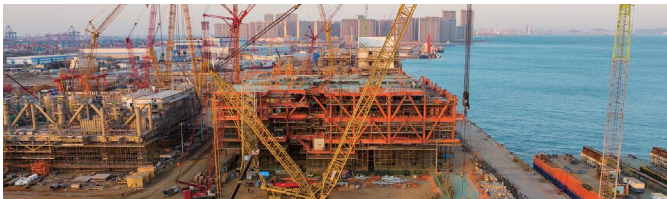
■ Onshore construction of modules of the Kenli 10-2 Project
