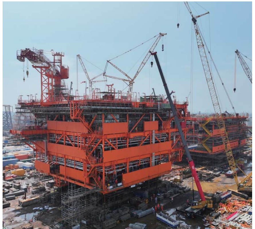
Onshore construction of the CEPE platform of the Bozhong 19-2 Oilfield Development Project
