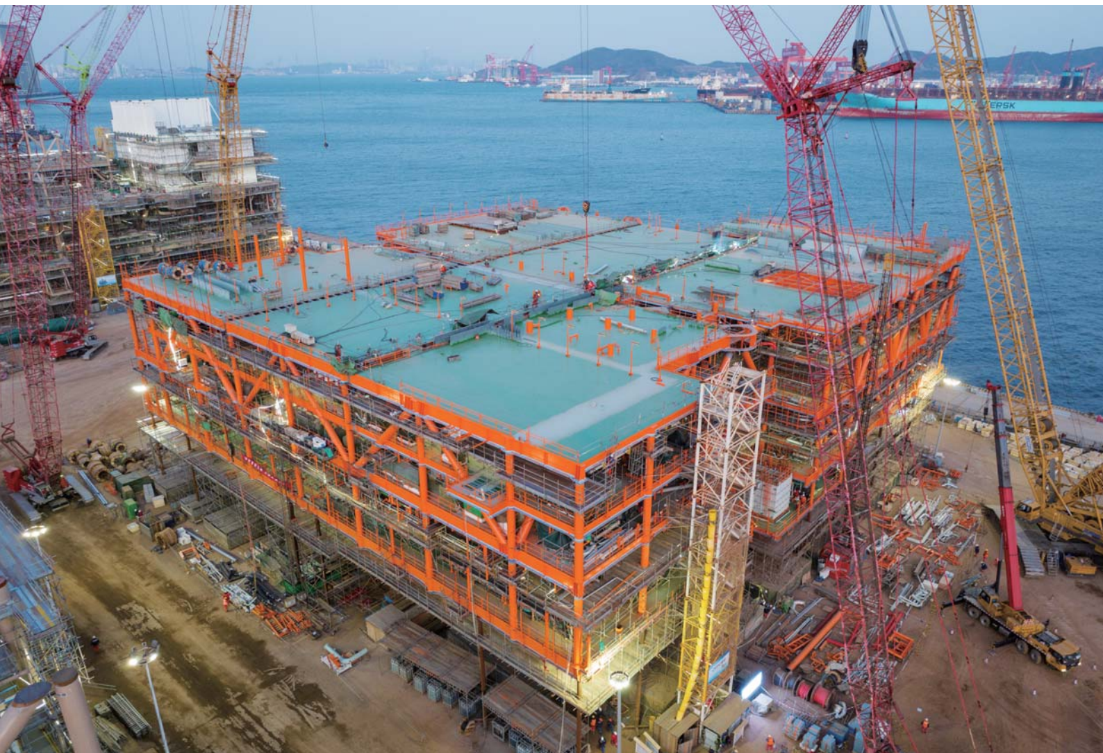
■ Onshore construction of modules of the Kenli 10-2 Project
