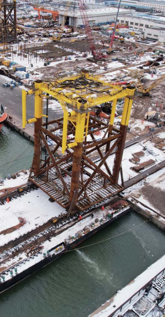
Onshore construction of the CEPE jacket of the Bozhong 19-2 Oilfield Development Project
