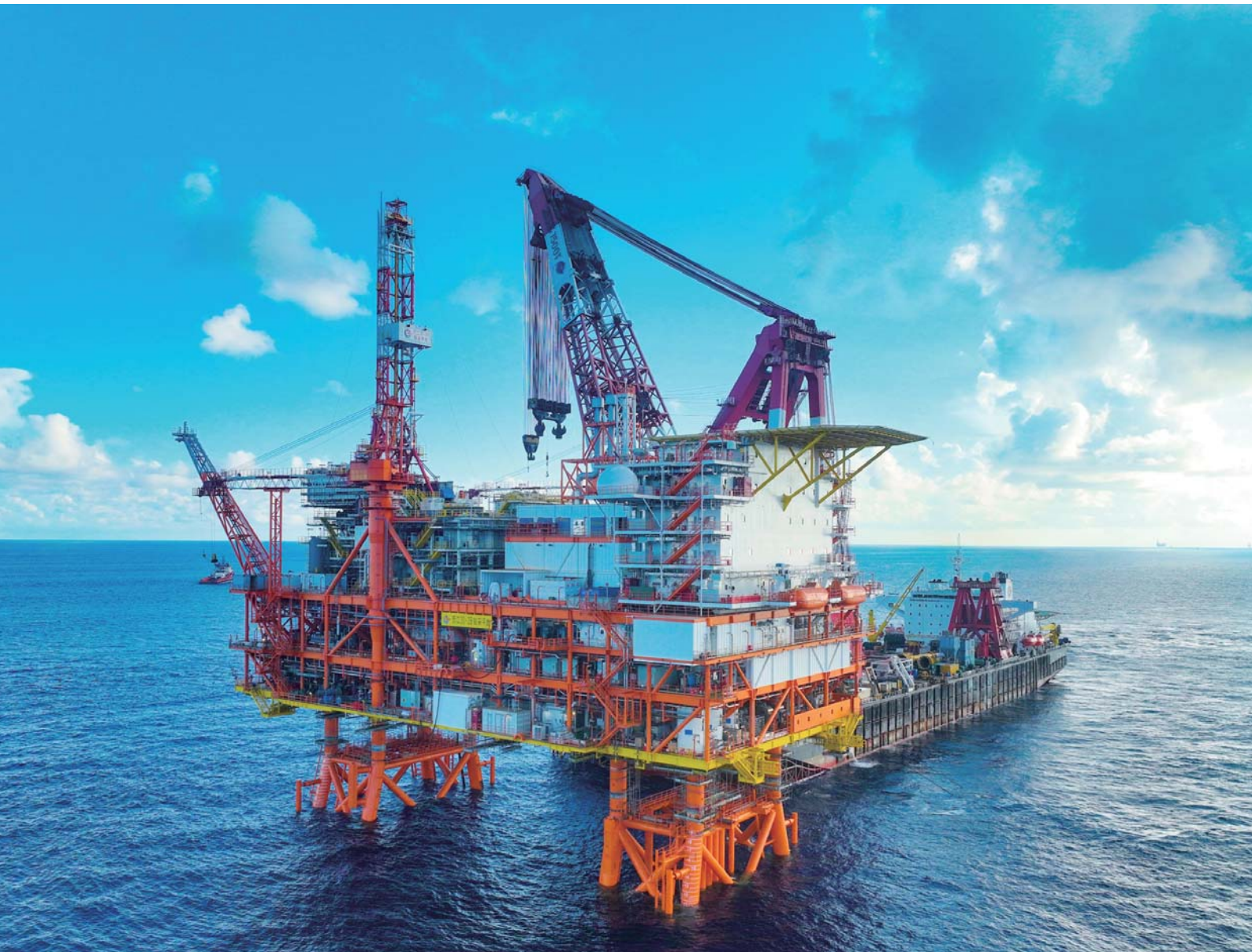
Offshore installation of the DPP B module of the Xijiang 30-2 Project
