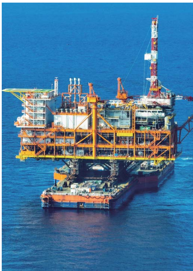
■ The "offshore oil 229" vessel of the Xijiang 30-2 Project with the topside module carried out the pre-installation procedure rehearsal of floatover operation
