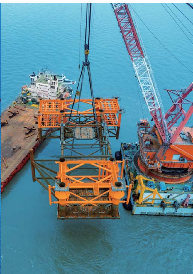
■ Offshore installation of the CEPA Jacket of the Jinzhou 23-2 Oilfield Development Project
