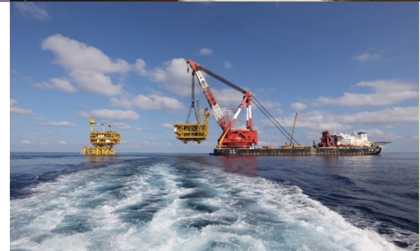
▲ Movement of Haiji-1 by Hoisting
