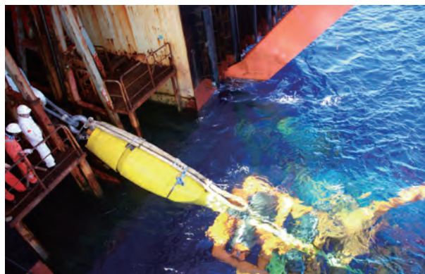
Launching of a pipeline end termination (PLET)
