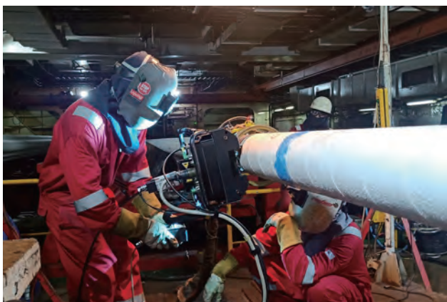
Welding of subsea pipeline
