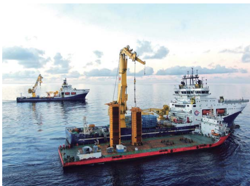
◀ Installation of Suction Piles with Offshore Oil 285 and Offshore Oil 287 Vessels
