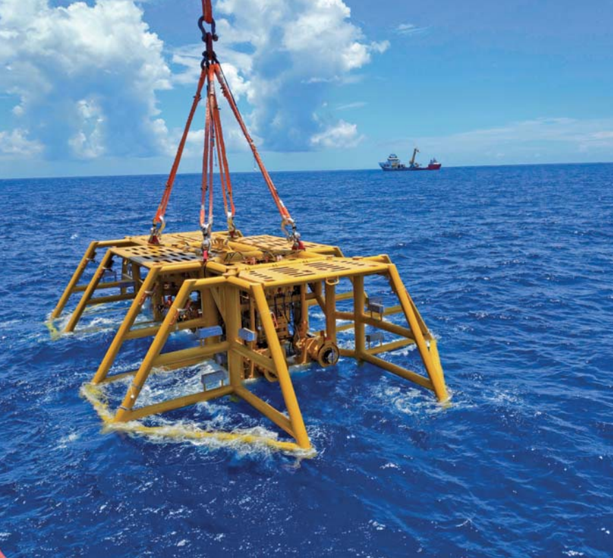
Subsea Manifold Installation of Lihua 16-2 Oilfield Group Project
