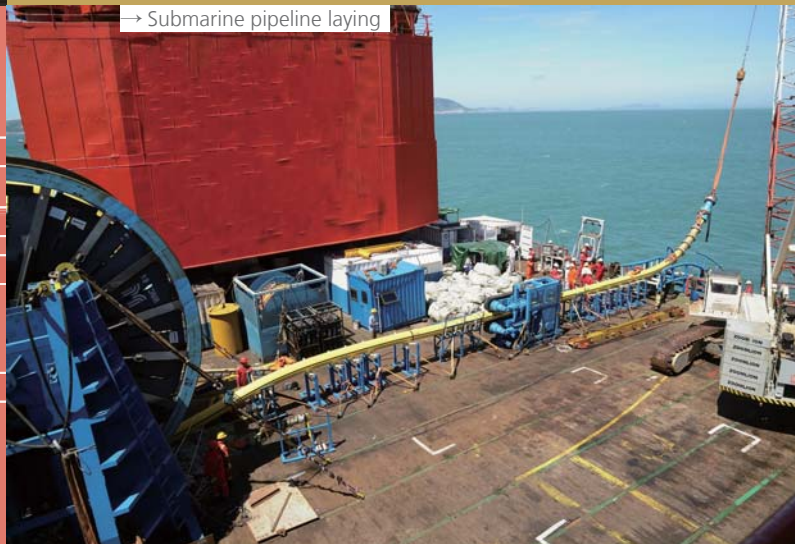
→ Submarine pipeline laying
