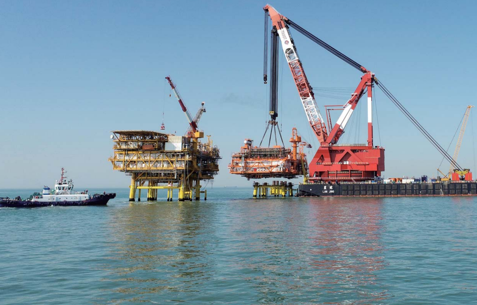
▲ Offshore installation of Bozhong 19-6 Condensate Gas Field Phase I Development Project
