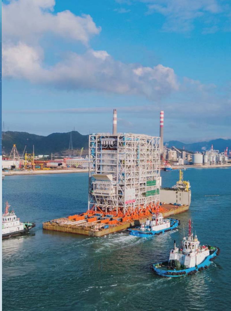
▶ Integrated module of Hong Kong Waste Power Plant Project
