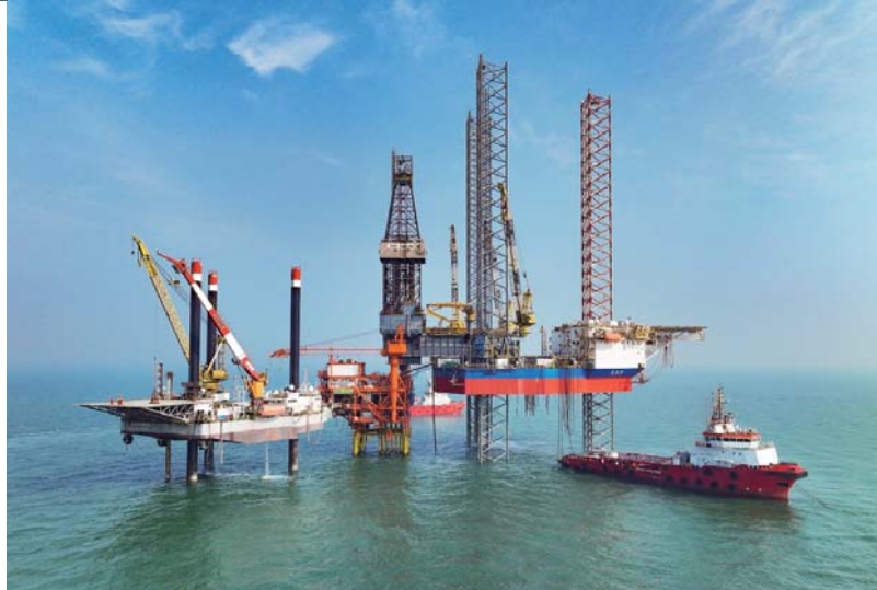
▶ WHPG platform for Development Project of Blocks KL5-1, 5-2 and 6-1 in Kenli 6-1 Oilfield
