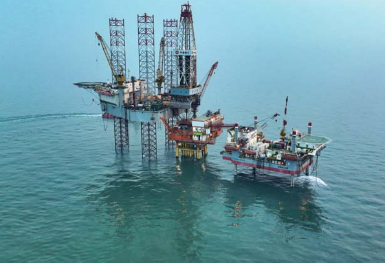
◀ WHPD platform for Development Project of Blocks KL5-1, 5-2 and 6-1 in Kenli 6-1 Oilfield
