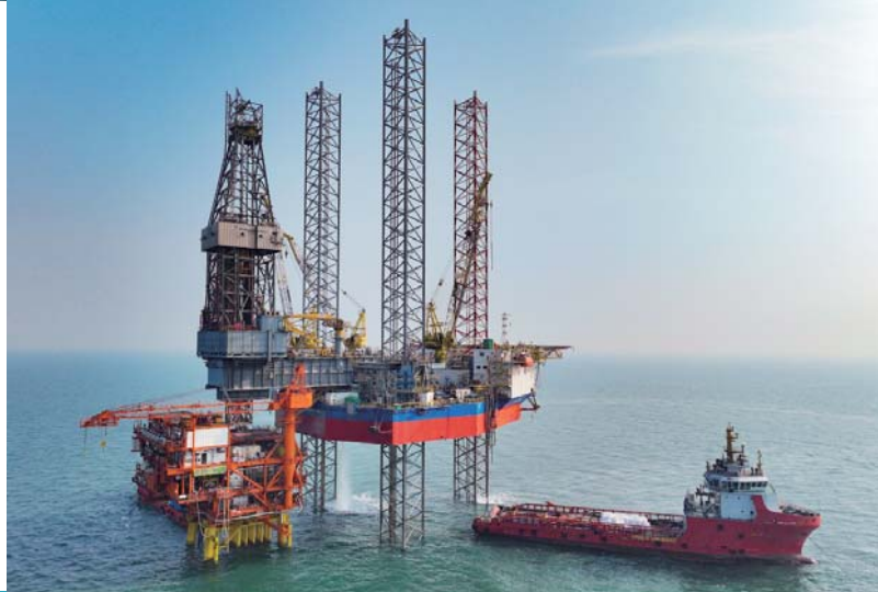
▶ WHPE platform for Development Project of Blocks KL5-1, 5-2 and 6-1 in Kenli 6-1 Oilfield
