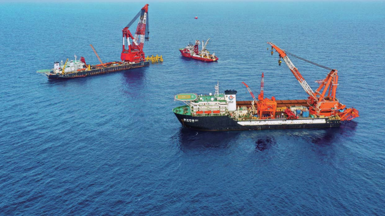
▲ Offshore installation of Lufeng Oilfields Regional Development Project
