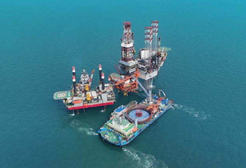
◀ WHPF platform for Development Project of Blocks KL5-1, 5-2 and 6-1 in Kenli 6-1 Oilfield
