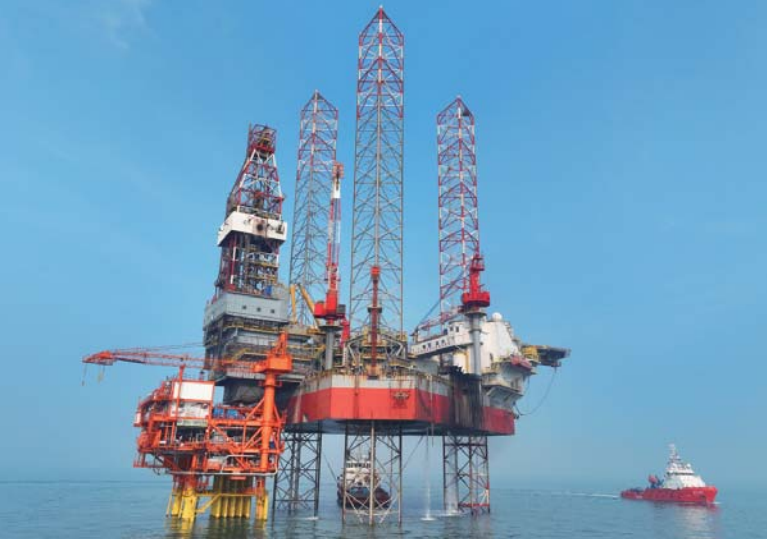
◀ WHPB platform for Development Project of Blocks KL5-1, 5-2 and 6-1 in Kenli 6-1 Oilfield
