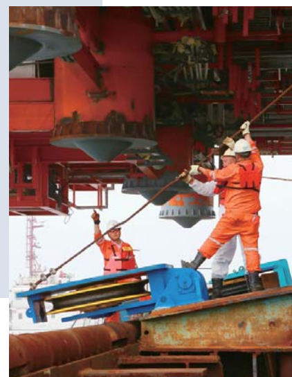
▶ Offshore installation site
