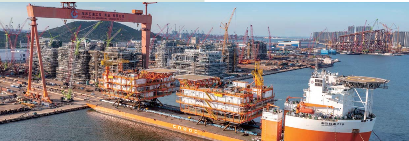
▼ Shipment of modules for Bozhong-Kenli Oilfields Shore Power Application Project
