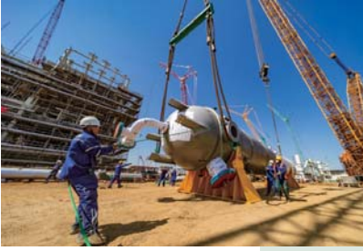
◀ Construction workers were working together to prepare for the hoisting operation
