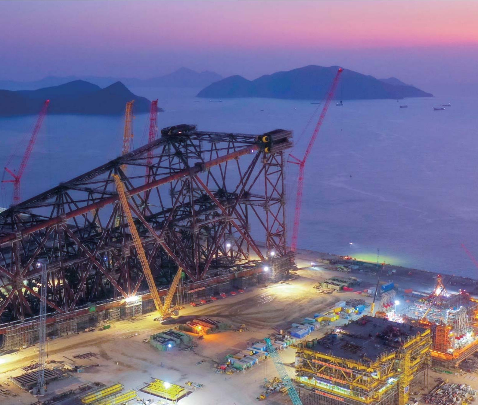
▼ Haiji-1 construction site of Lufeng Oilfields Regional Development Project
